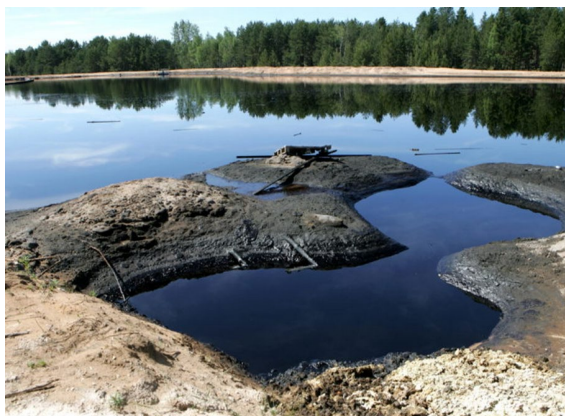
Fig. 1. A storage pond for “sour” sludge and “sour” water
